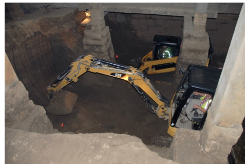
C. J. Moyna employees use a mini-excavator and skid loader inside the Motor Mill basement to remove sediment.
