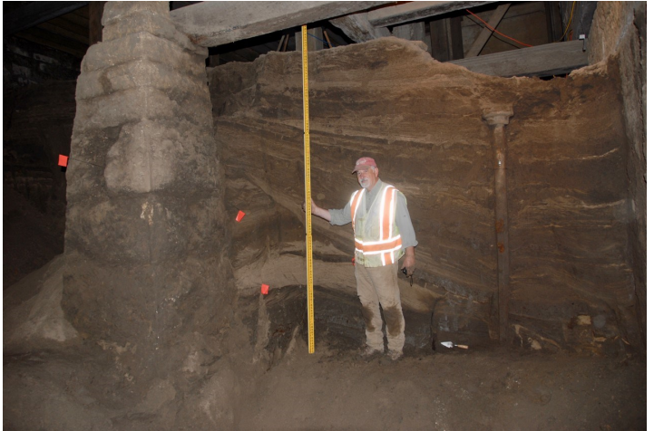
Retired archeologist Chris Schoen measures the sediment profile and the stone footings in the Motor Mill basement. Note exposed turbine shaft on right.
